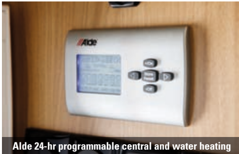
Alde 24-hr programmable central and water heating
